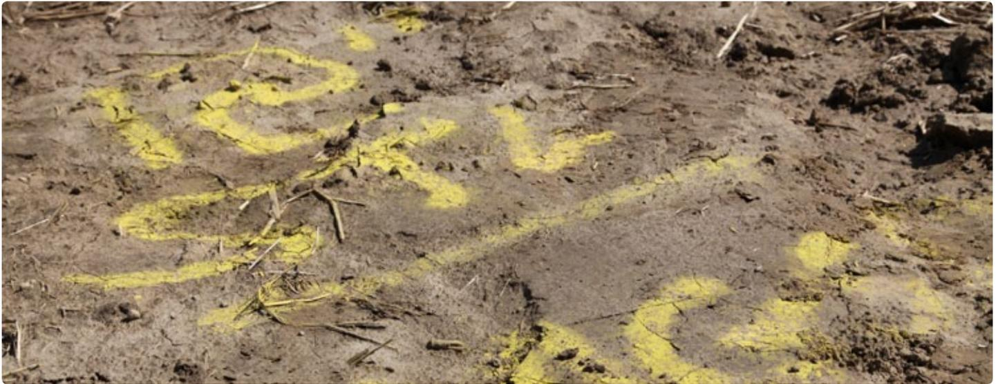
Temporary markings identify the location of an underground gas pipeline. Markings, like this one, communicate important information needed to work safely near underground infrastructure.
