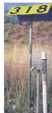
Front Range Pipeline, LLC Pipeline Marker Types
