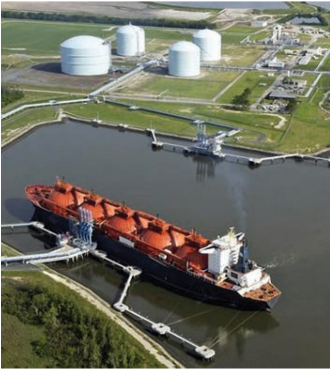
Insulated Low Pressure Storage Tanks for LNG
